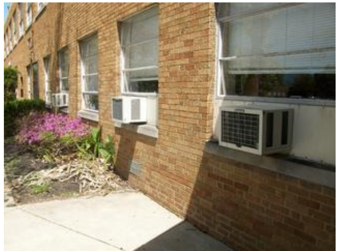
Window Air Conditioner Unit
