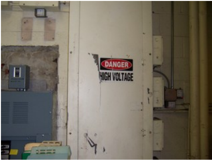
Original Building Main Electrical Panel
