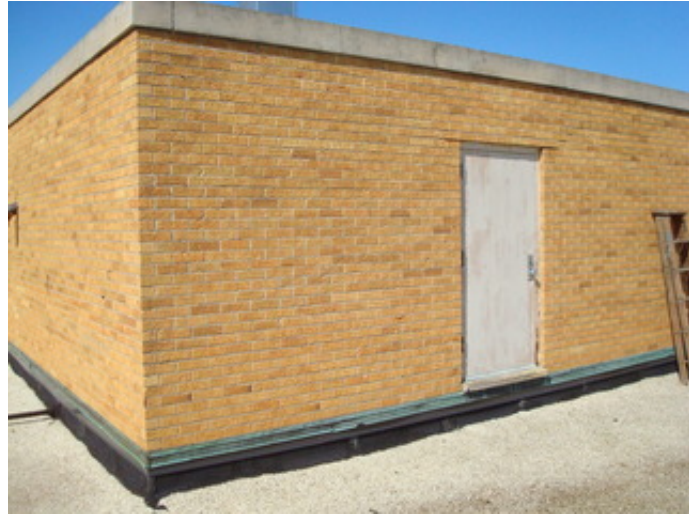
Damaged wall at 1970 Addition gymnasium
