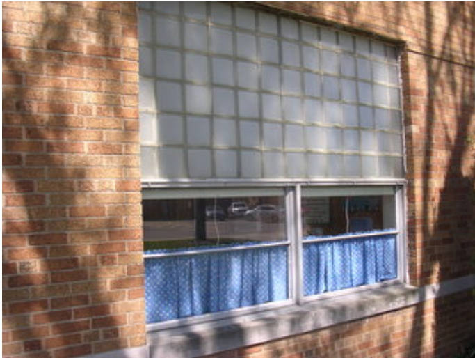
Typical aluminum windows with glass block.
