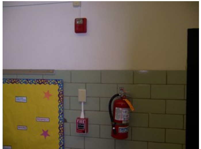
Typical Fire Alarm Devices
