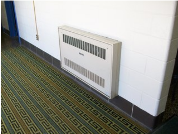
Typical Electric Unit Heater
