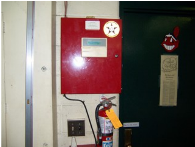
Fire Alarm Panel
