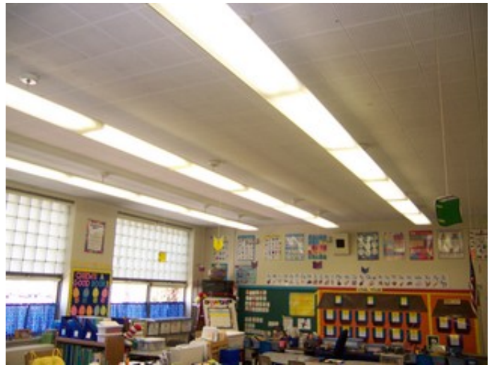
Typical Classroom Lighting
