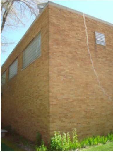
Damaged wall at 1951 Original Construction gymnasium
