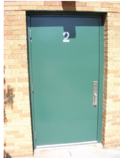
Typical hollow metal doors.
