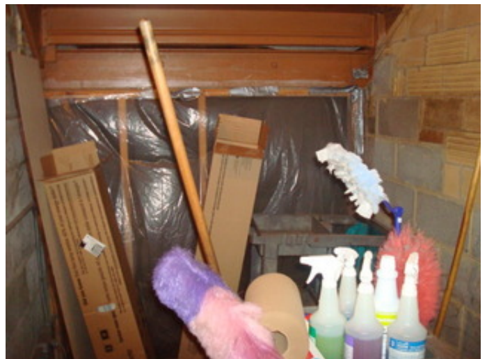
Encapsulated tunnel reported to contain asbestos
