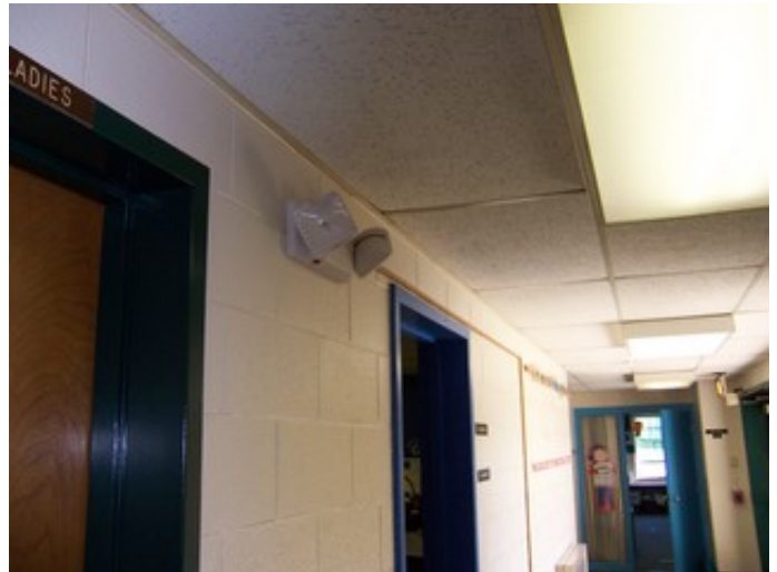
Wall Mounted Emergency Lighting
