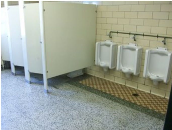
Toilet room fixtures
