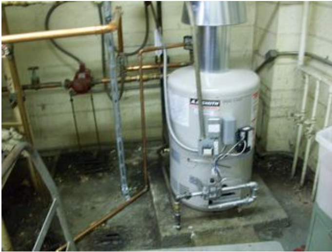
Domestic water heater
