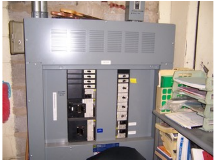
Electrical Distribution Panel
