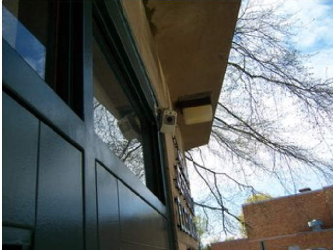
Main Entrance CCTV
