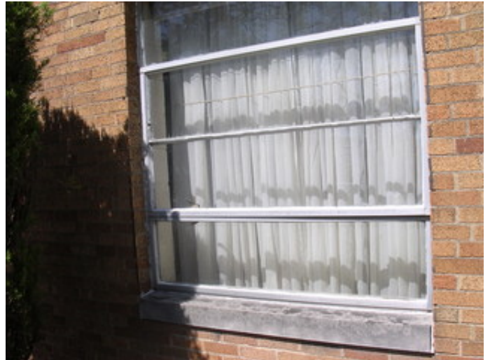
Typical aluminum windows.
