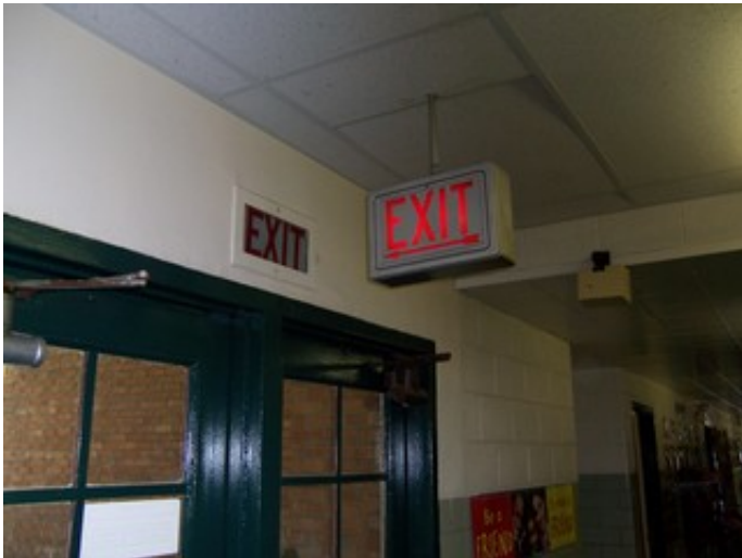
Emergency Exit Signs
