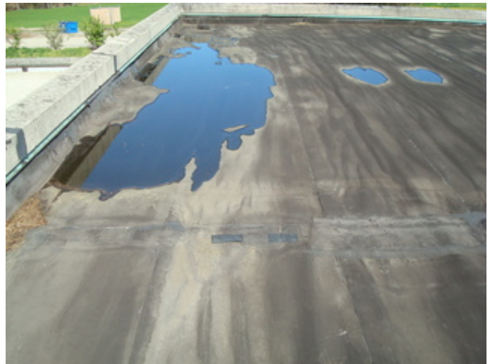
Patched area and standing water on 1970 Addition gymnasium
