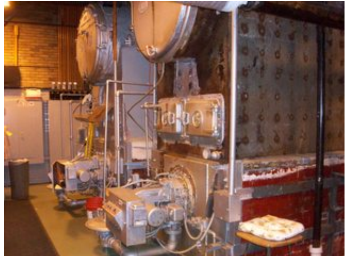
Gas Fired Boilers (At Eastlake)
