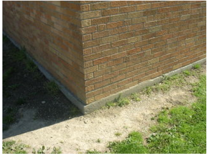
Typical exterior footing condition.
