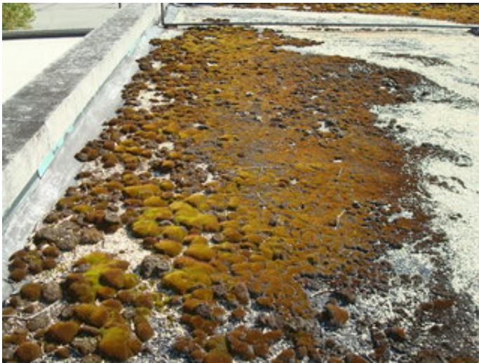
Significant moss growth on 1951 Original Construction
