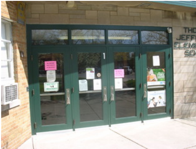
Typical hollow metal entry doors.
