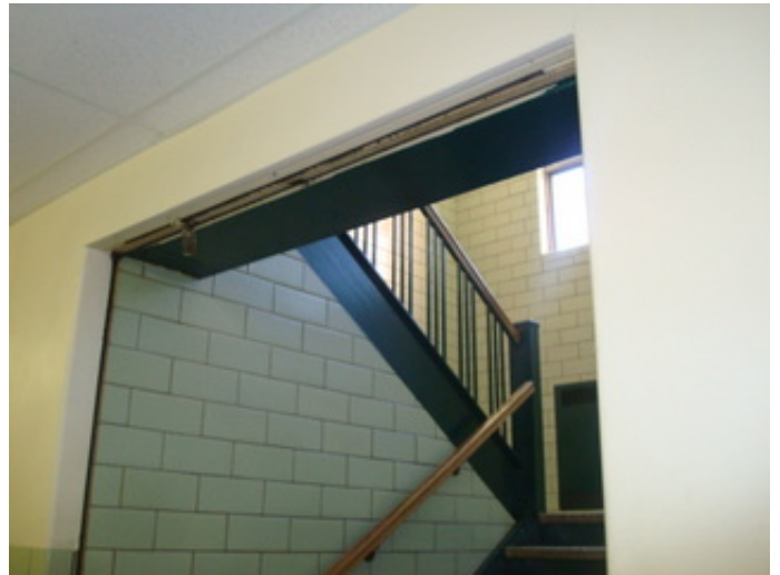
Stair guard and handrail
