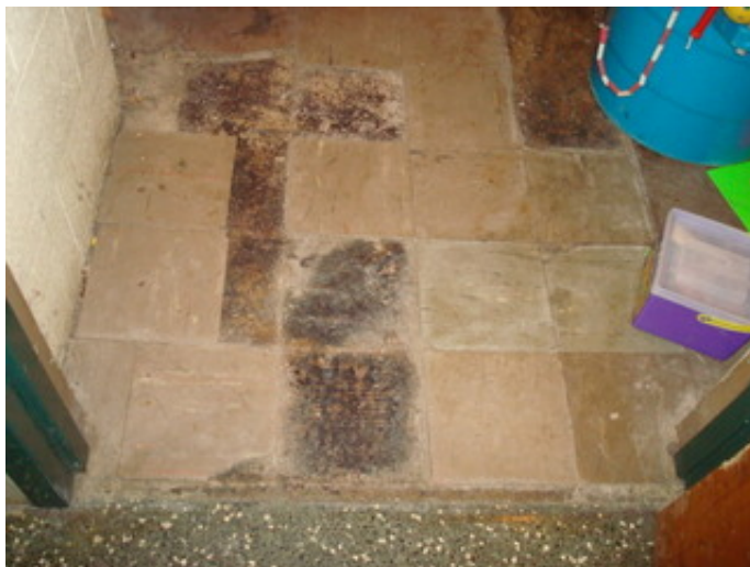
Vinyl tile in friable condition
