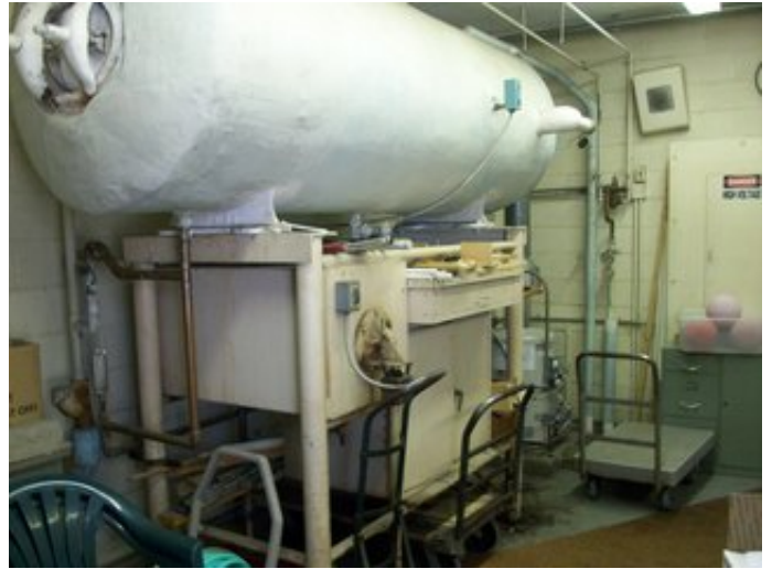
Storage tank and water piping
